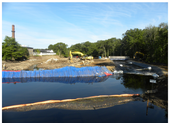
THE PAWCATUCK RIVER TEMPORARY RACEWAY LOOKING DOWNSTREAM FROM THE BRADFORD BRIDGE. BEHIND THE BLUE BARRIER IS THE DRY RIVERBED WHERE THE NEW FISH WEIR IS UNDER CONSTRUCTION.
